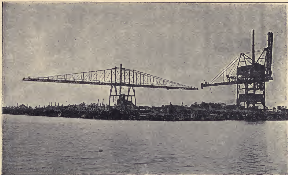
Pier 14 in the harbor of Cristobal.
